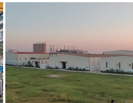
Akij Plastics Chhatak Plant (Bangladesh)
