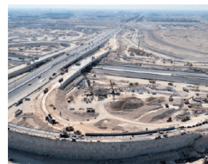
Al Khor Expressway (Qatar)
